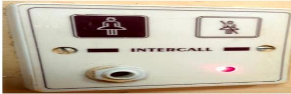
Figure (7) press on the button of “reset” in the master call point device to start over again
